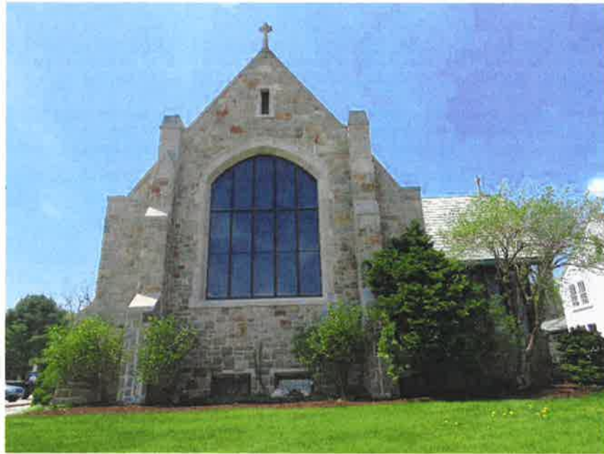
Photograph 1: The front of the church faces east toward Chestnut Street.
