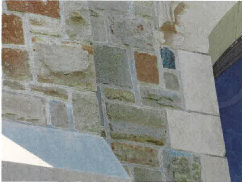
Photograph 5: The mortar is both light and gray in color.
