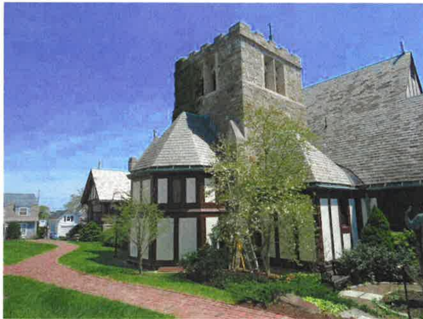
Photograph 2: The north (side) elevation of the church, the altar is north of the bell tower.
