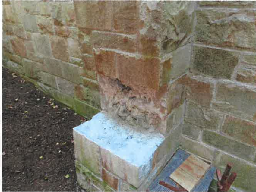
Photograph 13: Sections of the concrete on the north elevation is removed and being replaced.
